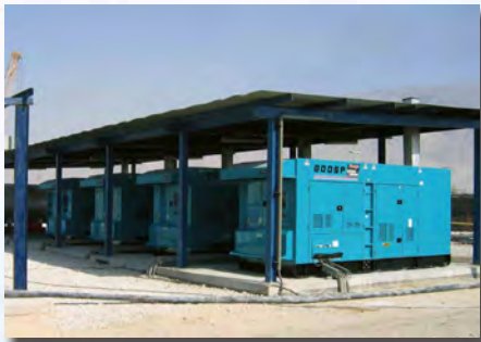
As the power source in the area where electricity is unavaible.
